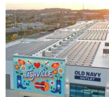
On-site solar energy production lowers our shared carbon footprint
